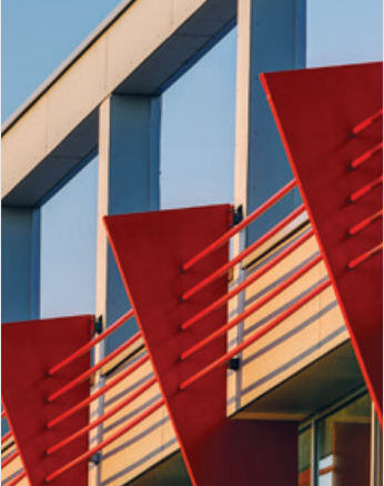
Exterior metal features on buildings
