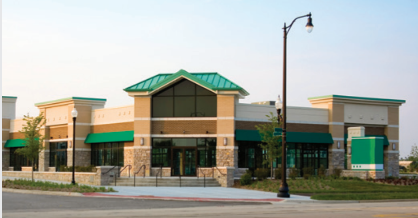
Light fixtures Signage
